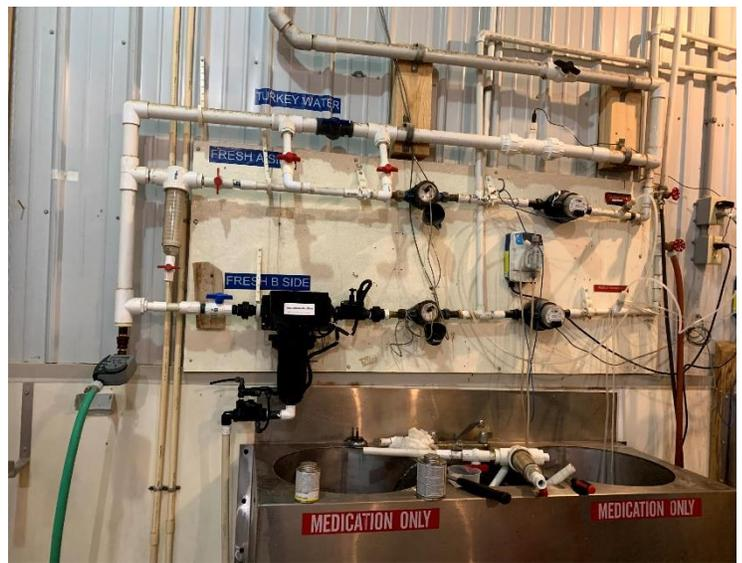
1" pipe, in-line livestock installation + drain
